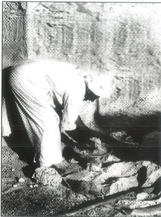
A Mason while preparing «qeela», i.e. the mud and placing it in the pan to hand it over to al astad.
