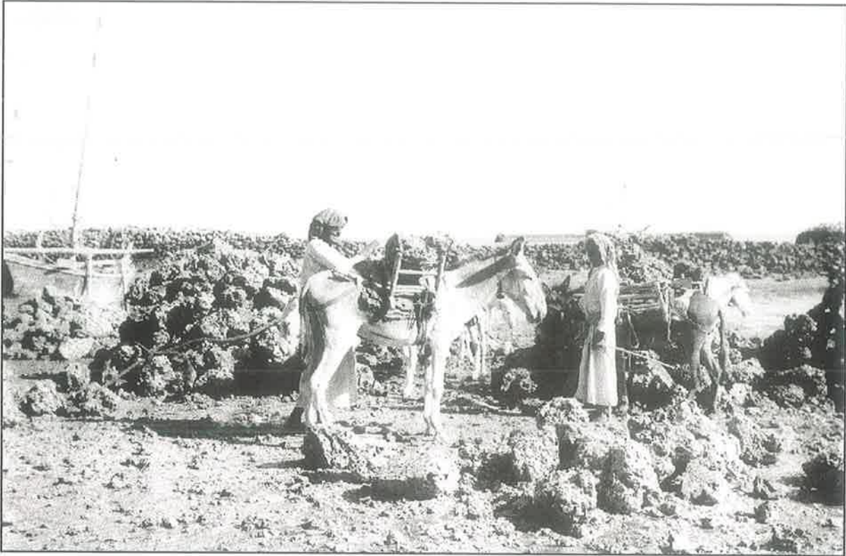
Donkeys were used for carrying rocks from the niq'a to the building locations. Rocks were brought from O'shairej through «tashasheel» which unloaded them at the niq'a in the form of piles.
