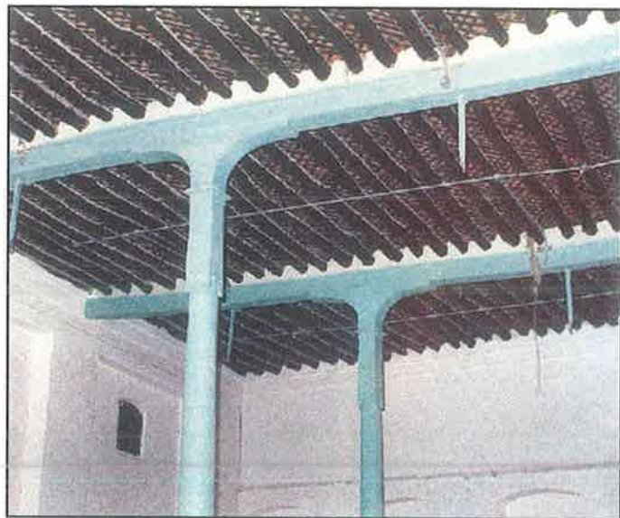
The roof of an ancient mosque. Two sowars «beams» are seen while carrying al chandal upon which the roof is based.
