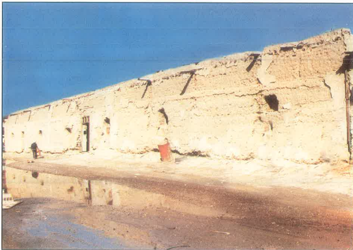
The wall of one of the old houses made of mud bricks
