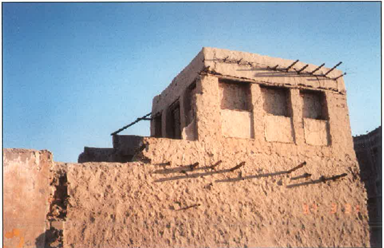
A two-floor house. The upper room is seen with ventilations known as «bagdeer».
