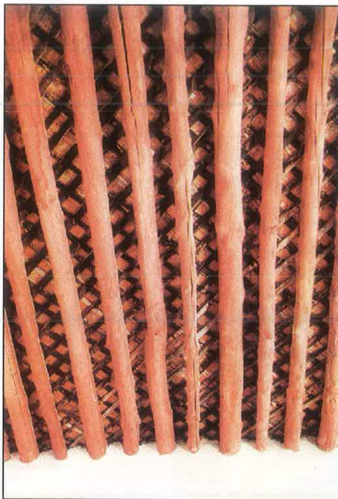
Room ceiling composed of bascheel, chandal and bawari
